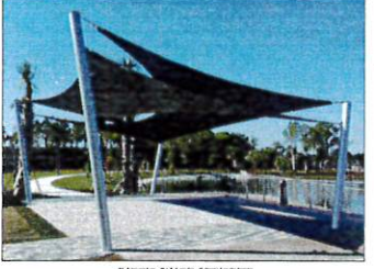
FABRIC SHADE STRUCTURE
